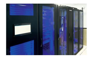
connection points. The Mini Data Centre supplied to the hospital is an all-in-one system with integrated climate control, energy distribution, uninterruptible power supply (UPS) as well as intelligent environmental, monitoring and management systems. It comprises five racks and a precision inrow cooler and is a completely closed system, so in that respect is very energyefficient.
